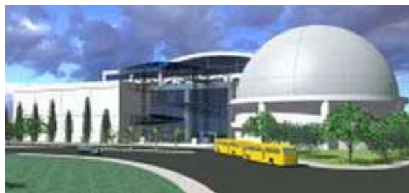
Photo: Perspective of the new Philippine Science Centrum, with state-of-the-art amenities and intelligent building features
